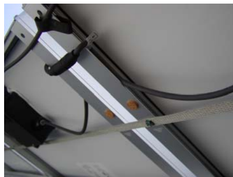
Figure 4 (correct) Shows continuous grounding strap
