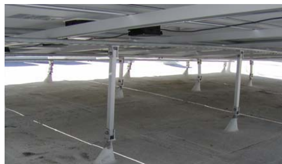
Figure 9 Flashed Penetration (correct)
