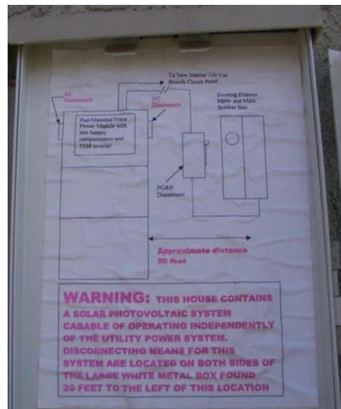
Figure 14 Close-up of sign for emergency personnel
