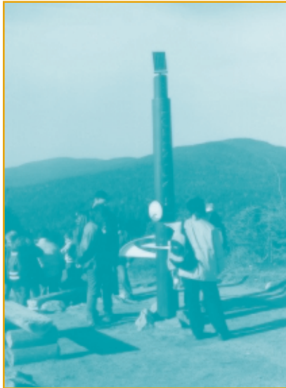
▲ A small PV module is used to power a trail indicator at night at Mont-Tremblant, Quebec. Photo courtesy of TN conseil inc.
