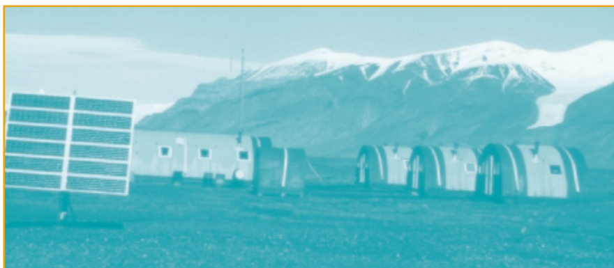
◀ Parks Canada's remote camp located in the far north on Ellesmere Island, Nunavut, is powered by a PV array (on a tracker) combined with a wind generator and a gasoline generator.
