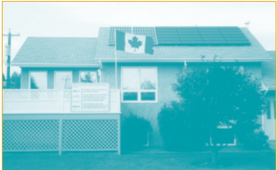
▲ This house in Edmonton, Alberta, is equipped with a 2.3-kW system that is connected to the local power utility. About 2500 kWh are produced each year. The investment cost in 1995 was $28,000.
