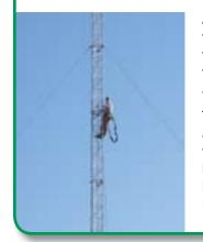
A wind generator tower is very often more expensive than the turbine. The tower puts the turbine up in the "fuel" the smooth strong winds that give the most energy. Wind turbines should be sited at least 30 feet (9 m) higher than anything within 500 feet (152 m).
